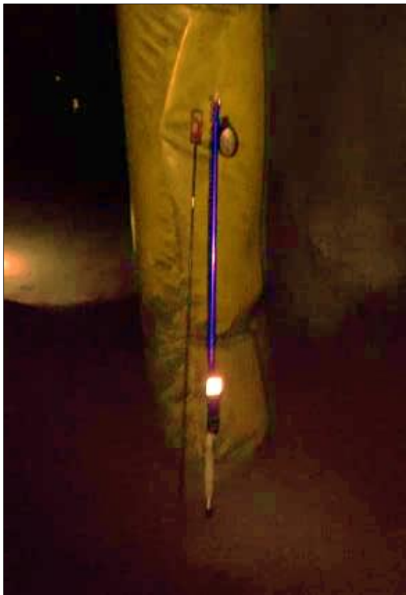
Figure 16-21: Safescape Zipper Jacket at Base of Ladderway
